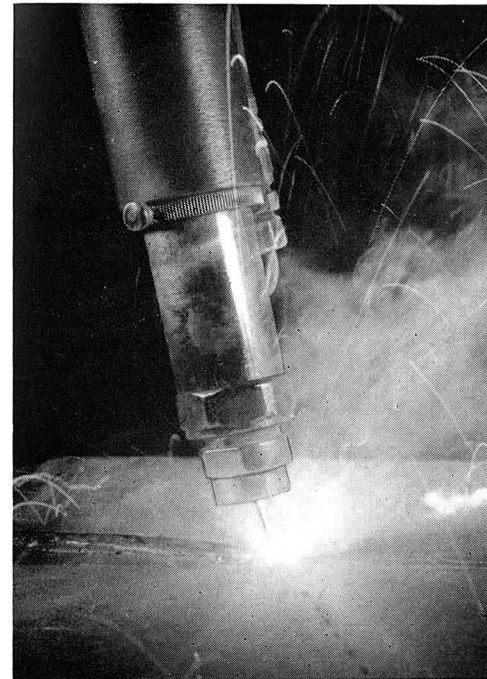
Carbon dioxide welding of 1" thick mild steel
